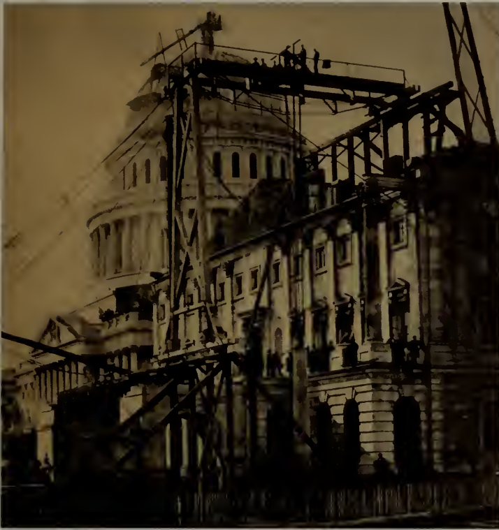
A marble monolithic column for the Senate portico is swung into place. In the background the dome nears completion.
